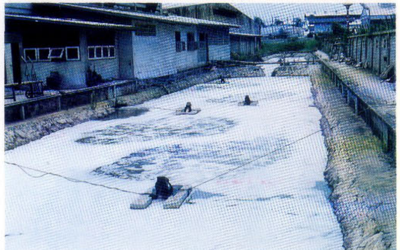
The horizontal aeration technic offers mixing capability unmatched by other aeration system.
